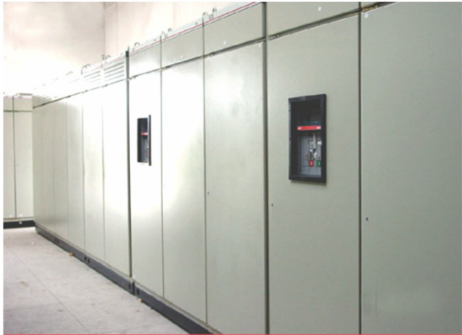
Cabinet with GB ARM low-pressure sealed cabinet or similar standard products like GGD cabinet shell
